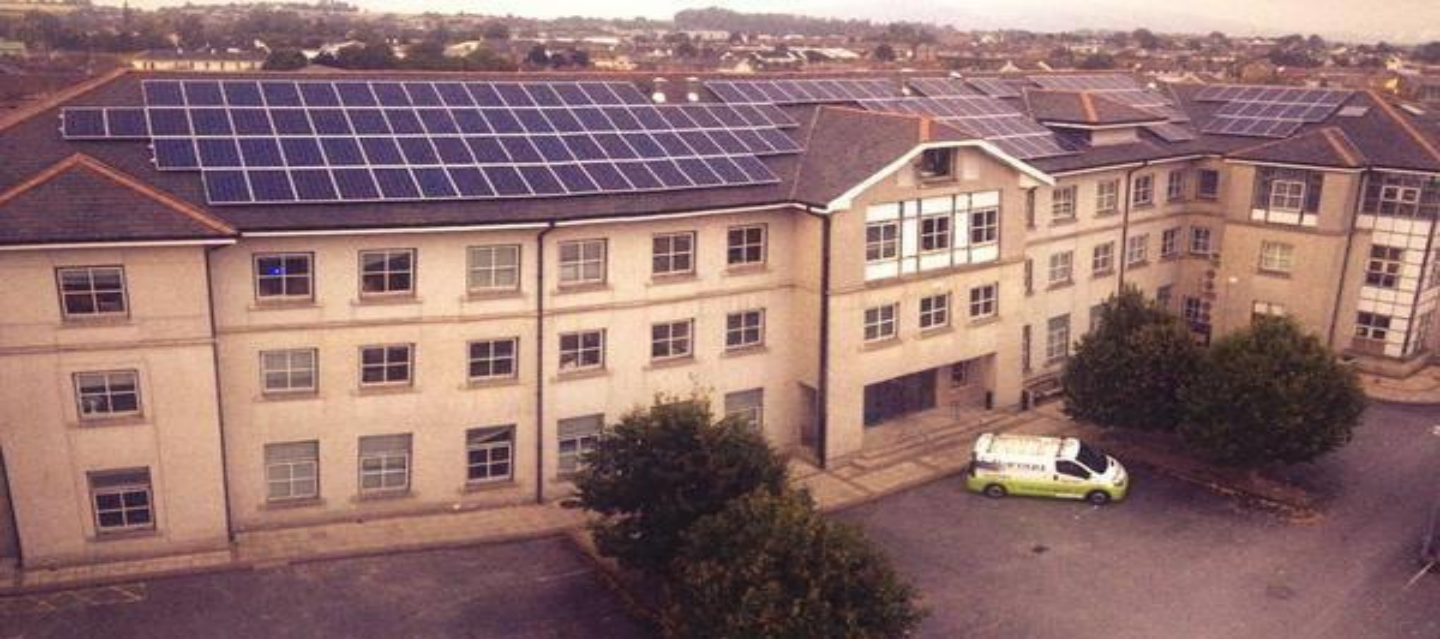
Ireland's largest Solar PV installation, County Hall Clonmel, Tipperary
